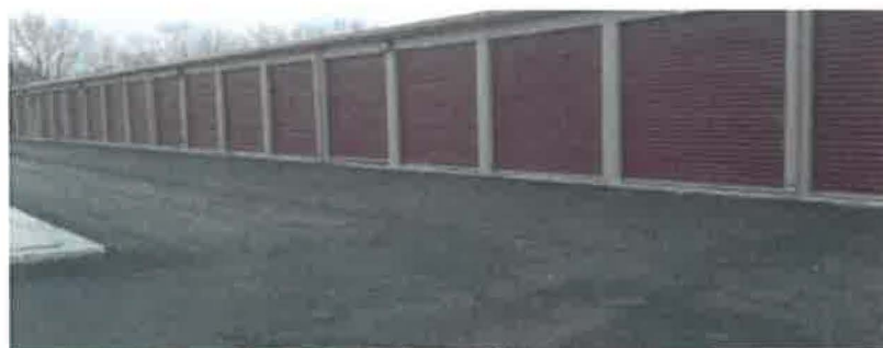
Example of Self-Storage Facilities having numerous garages.
